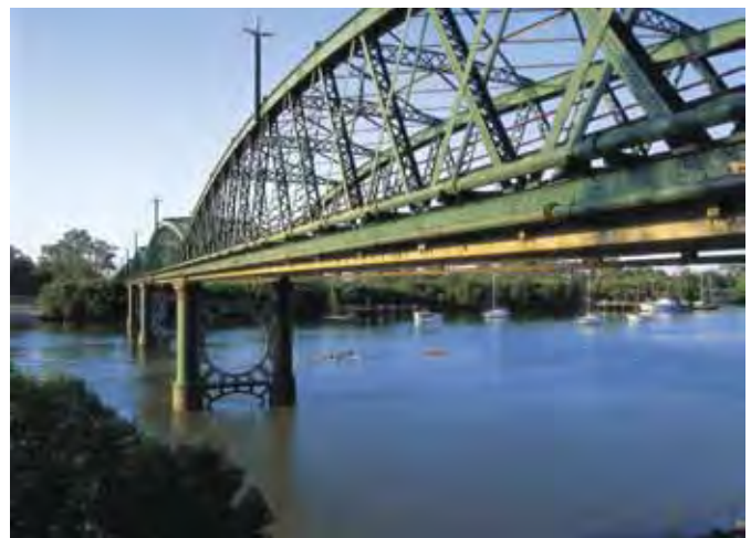
Burnett River Bridge, Bundaberg Courtesy of Murray Waite & Assoc
